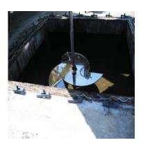
The Clean Edge impeller pictured left remains free of fibrous debris while delivering performance equal to a hydrofoil impeller.
