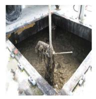
Pictured to the left is an Anoxic Mixer at a WWTP in Florida. The hydrofoil impellers installed here bind up with rags and other fibrous materials until the blades, shaft or mixer drive require maintenance and/or replacement.
